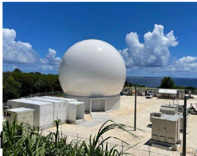
The new TT&C station at Miyakojima-island
