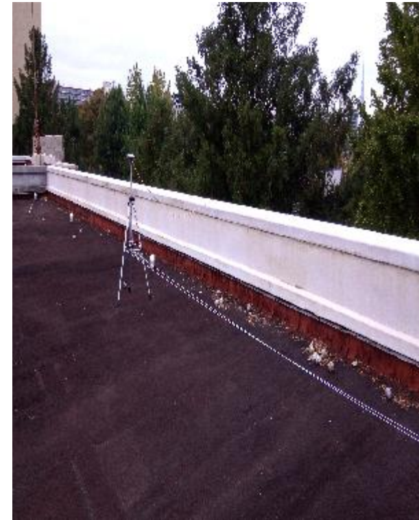
Temporary base station
